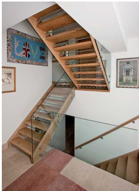
Oak open riser stairs with 15mm toughened glass, no handrail required for this type of stairs
