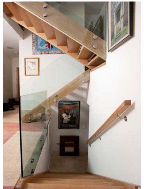
Oak open riser stairs with 15mm toughened glass, no handrail required for this type of stairs
